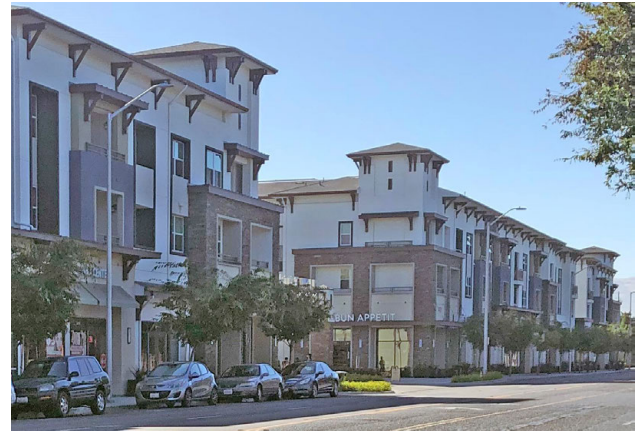
Mixed-use development with bracket details at the cornice and roof eaves; ground floor height of at least 15 feet high; and distinct top, middle, and base.
