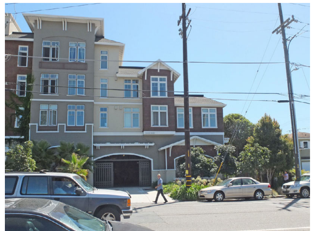
Multi-family residential building height stepped down near adjacent single-family residence.
