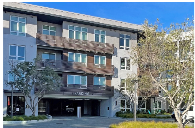
Multi-family residential project with podium parking on the ground floor.
