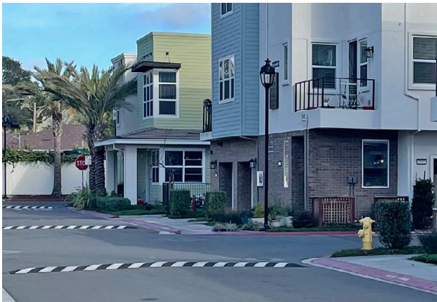
Internal street within a townhouse development leading to an alley with access to garages.
