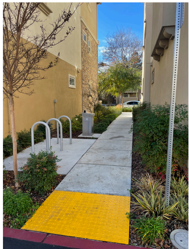
Pedestrian walkway connecting the public sidewalk to residences with bicycle parking.
