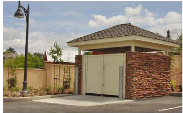
Trash area screened from public view, covered with a roof, and located to provide access to service provider vehicles.
