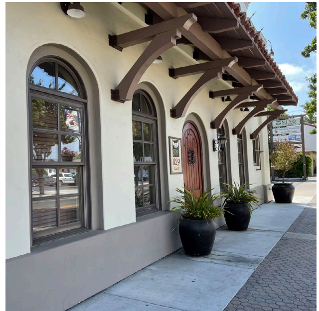
Recessed, vertically oriented and proportioned windows with true divided lite divisions on a street-facing facade.
